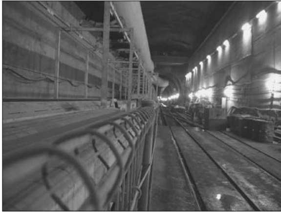
Figure 4. Adit 10 TBM assembly and materials handling chamber
