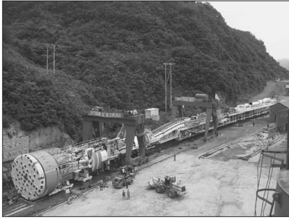
Figure 5. TBM3 at downstream portal
