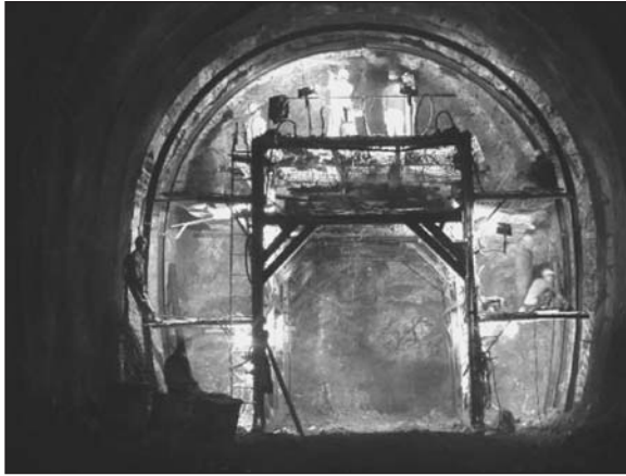
Figure 7. Drill + shoot platform jumbo
