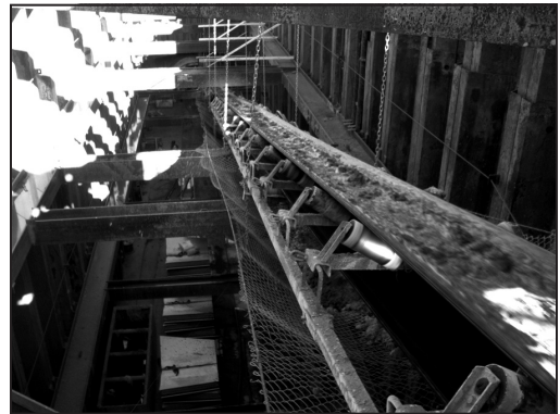
Figure 2. Conveyor system with consolidated muck and additive: UNWI Project, Sacramento, CA
