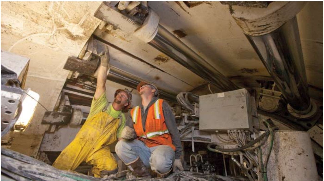
The 4.25 m (13.9 ft) Robbins EPB is using concrete segments embedded with PVC inner liner to prevent corrosion by sewer gases.
