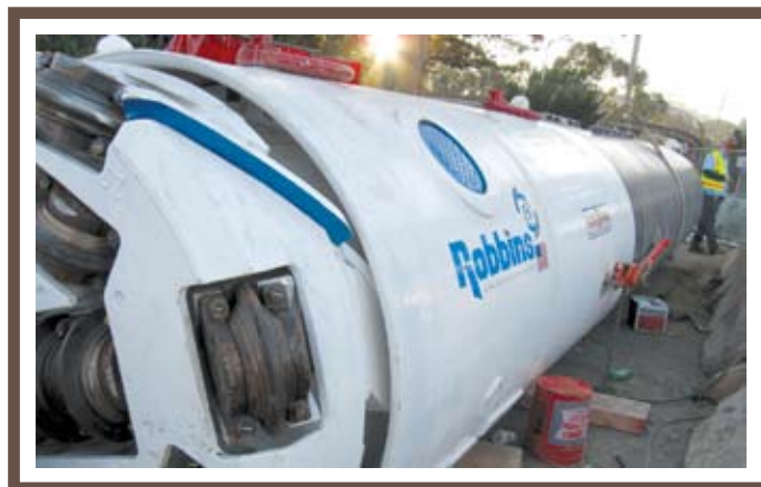
Left: The 1.5 m (60 in) Robbins Motorized SBU needed to bore 21 m (70 ft) in 72 hours. Middle: The 90 m (300 ft) long crossing undercut both rail tracks and a highway in San Francisco, USA. Photo: Steve Gallyer Bottom: The Robbins SBU-M made the deadline and completed the crossing by March 16, 2009.
