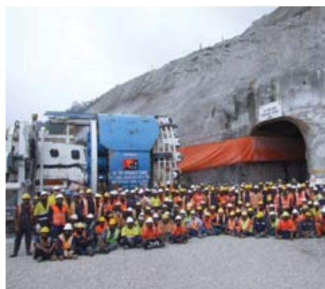
The 5.6 m (18.4 ft) Main Beam TBM was launched in late August 2008 in Papua New Guinea.
