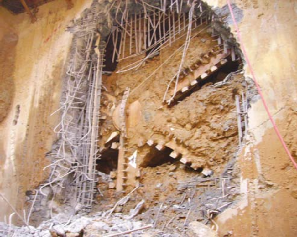
Left: The first 6.5 m (21.4 ft) diameter EPBM broke through on September 29, 2008. Above: The Robbins machine achieved advance rates of up to 19 rings per day.
