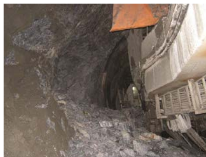
Figure 4. Example of rock bursting.
