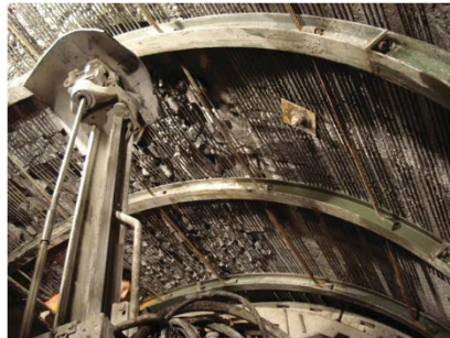
Figure 2. Detailed view of the McNally Support system.
