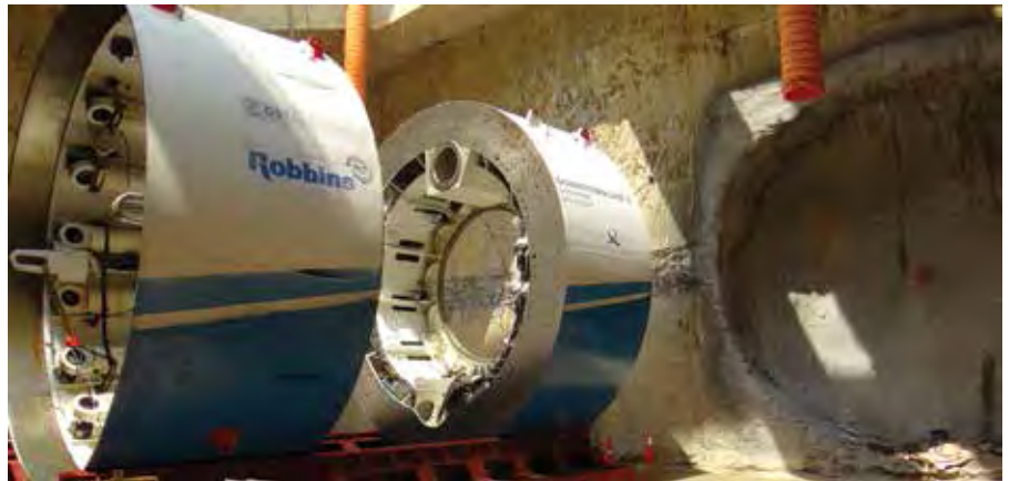
Above: Assembly of GS Engineering’s C925 EPB took place in a cradle that had to be jacked into place for the tunnel alignment.
