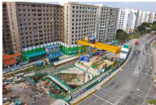
Above: The first of the five Robbins EPBs broke through at the C927 site in October 2013 after achieving advance rates up to 15 m per day.
