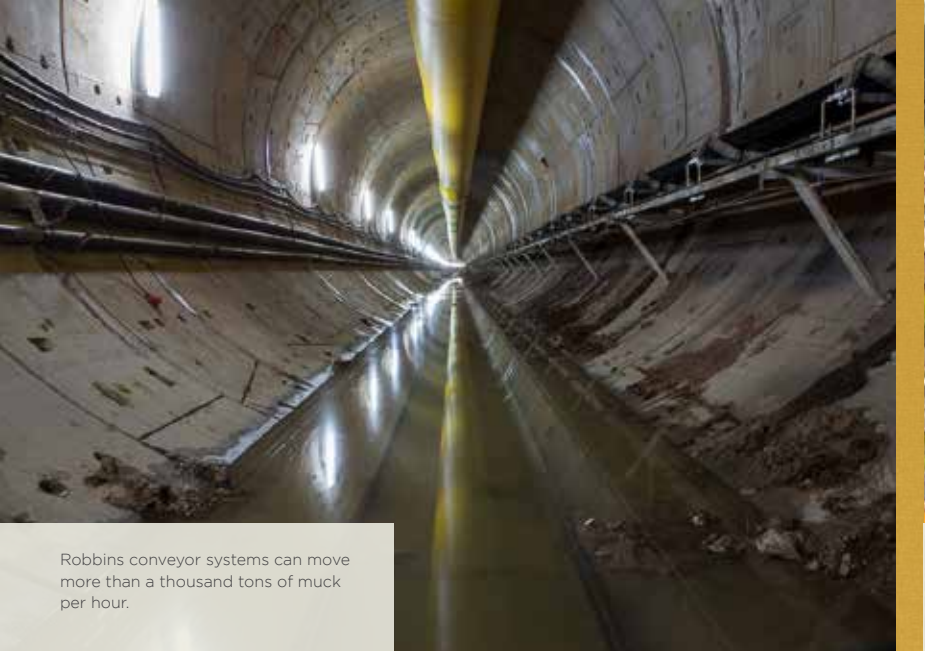
Workers inspect the Robbins continuous conveyor system operating behind a Crossover TBM at the TEP II jobsite in Mexico.
