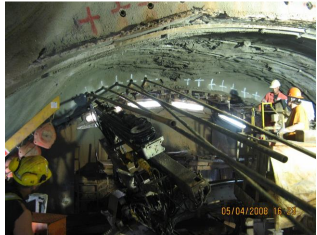
Figure 8. Forepoling on Main Beam Machine
