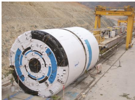
Figure 2. Double Shield TBM for somewhat fractured rock
