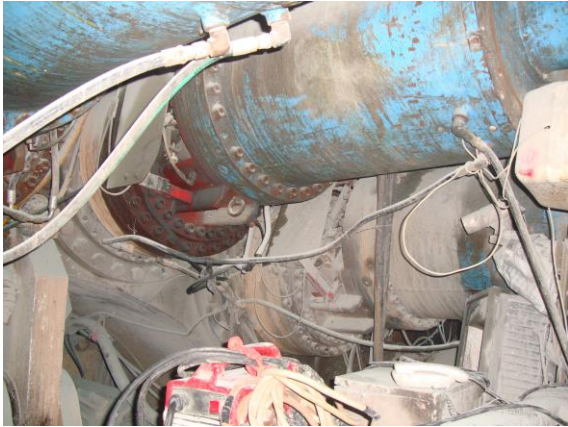
Figure 13. Two-speed gearboxes (red) installed on a Robbins Double Shield TBM
