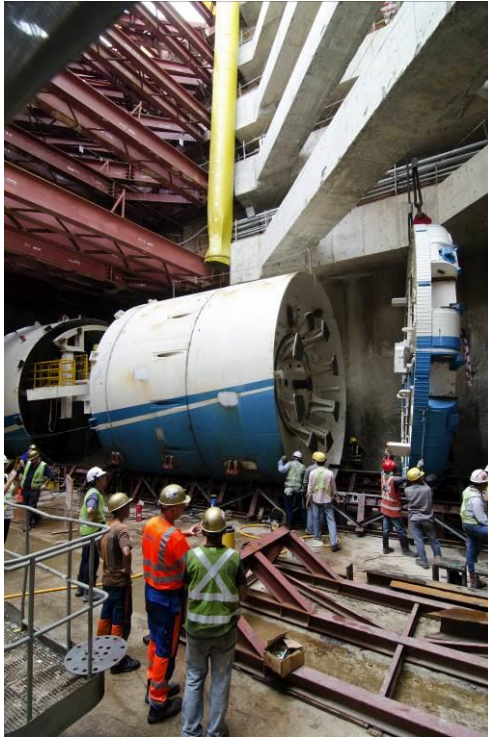
Figure 12. Assembly of one EPB on the C927 contract.
