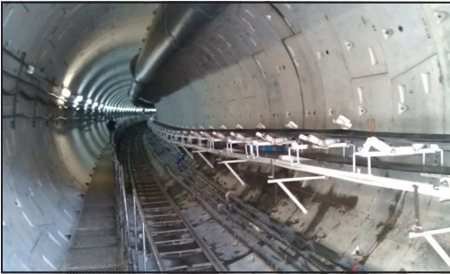
Figure 8. Horizontal conveyors going around a curve
