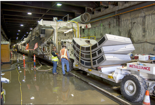
Figure 9. RTV transporting segments (Image credit: sfmta.com)
