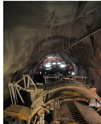
Figures 3 and 4. Overbreak – Niagara Tunnel Project.
