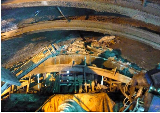
Figure 7. Roof collapse
