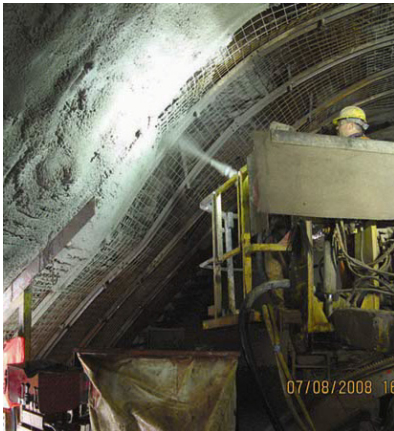
Figure 2. Shotcrete application
