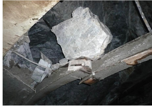
Figure 8. Ring beam failure
