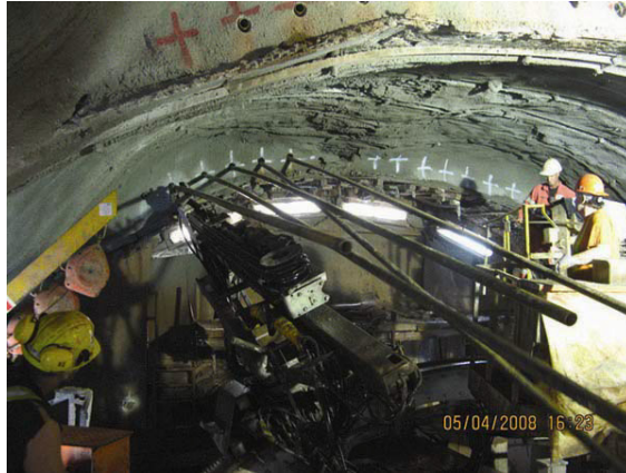
Figure 5. Spiling in Difficult Geology
