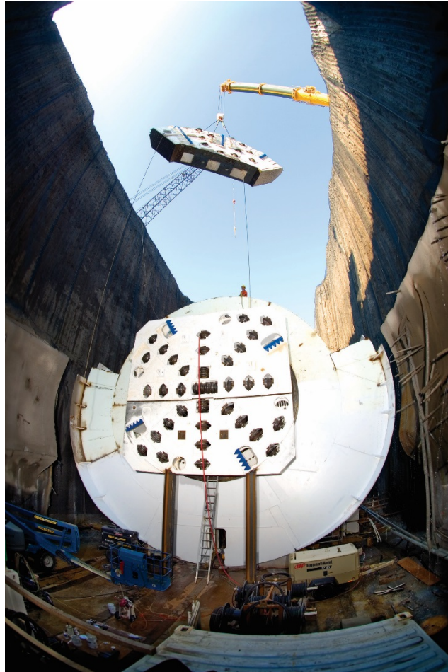
Plate 1: An example of Onsite First Time Assembly, Niagara Tunnel Project, Canada
