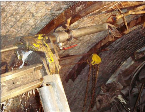
Figure 8. Drilling through stand pipe at Parbati
