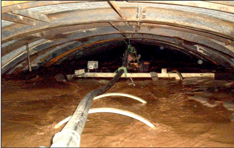
Figure 9. Parbati TBM buried in silt
