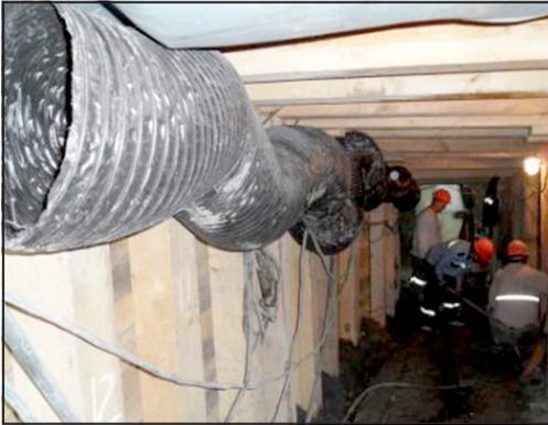
Figure 3. Bypass tunnel excavation
