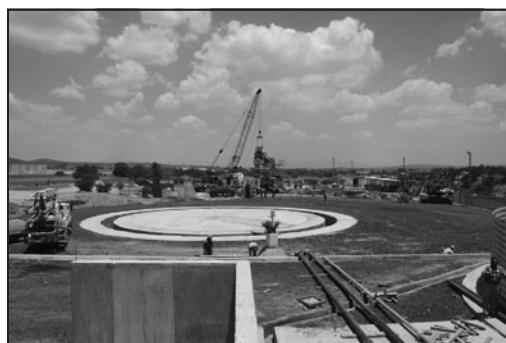
Figure 11. Slurry wall construction, Shaft 20, November 2009
