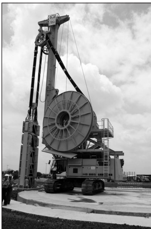
Figure 12. Hydro excavator machine, shaft 20
