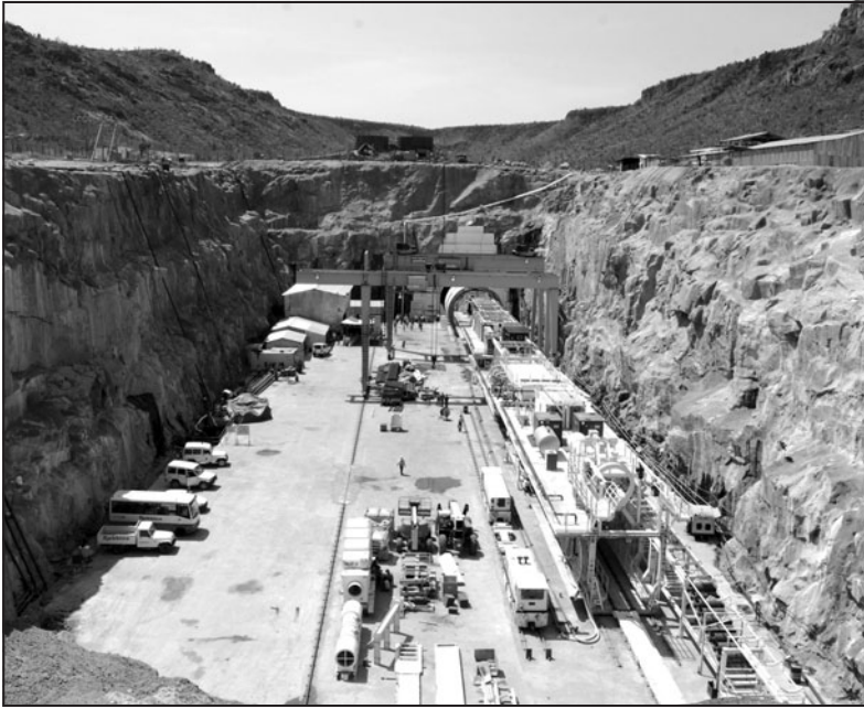
Figure 7. Assembly proceeding in the granite open cut
