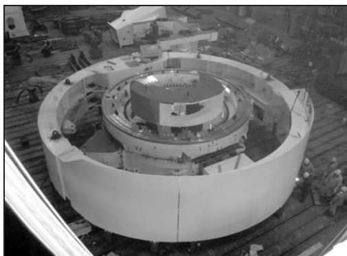
Figure 10. Pre-assembly of the cutterhead support and shields—Jin Ping II, China
