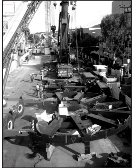
Figure 15. Assembling cutterhead sections with pedestal—Mexico MX12
