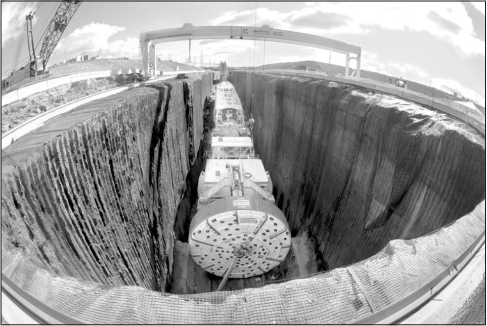
Figure 5. TBM and back-up assembled in launch chamber
