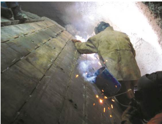
Figure 14. In-tunnel install of the McNally system
