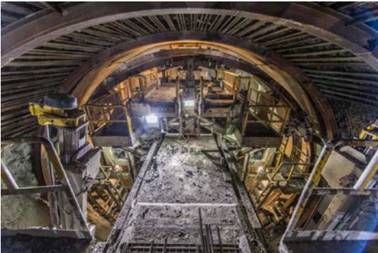
Fig. 8. McNally slats installed in the tunnel crown at Liaoning T5
