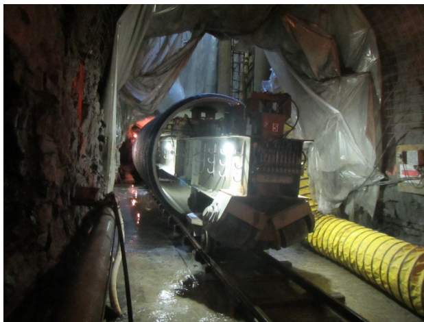
Figure 4. Pipe carrier with section of pipe
