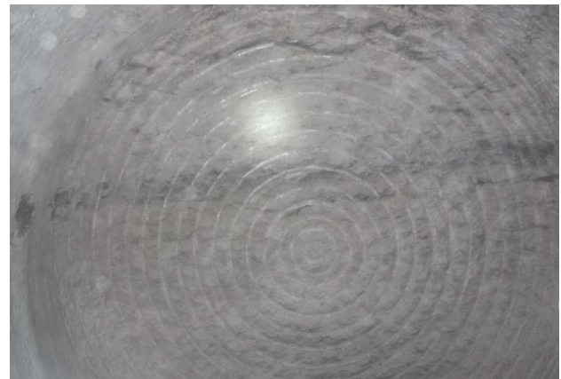
Figure 6. Example of the cutterhead "kerf" or cutting pattern
