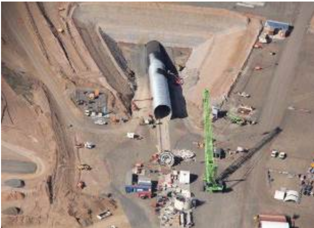
Fig. 16. Aerial view of the assembly area and decline launching tunnel
