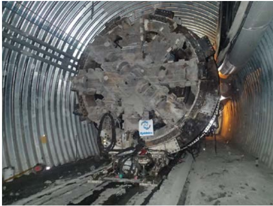
Fig. 11. TBM core retraction with transport dollies through the Conveyor Drift launching tunnel (July 2014)
