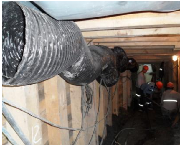
Figure 2. Bypass tunnel excavation.
