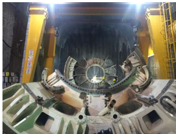
Figure 13. Assembly of the Gerede TBM in an underground launch chamber.
