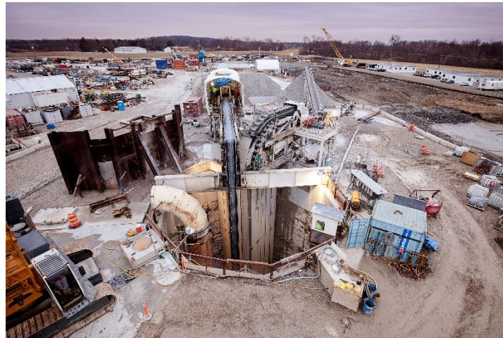
Figure 4. Setup of the conveyor system at the launch shaft
