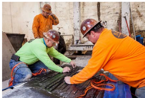
Figure 5. Crews vulcanizing a belt splice in Indianapolis
