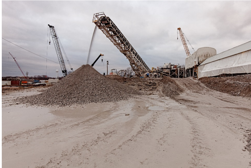
Figure 6. Stacker conveyor for temporary storage of muck
