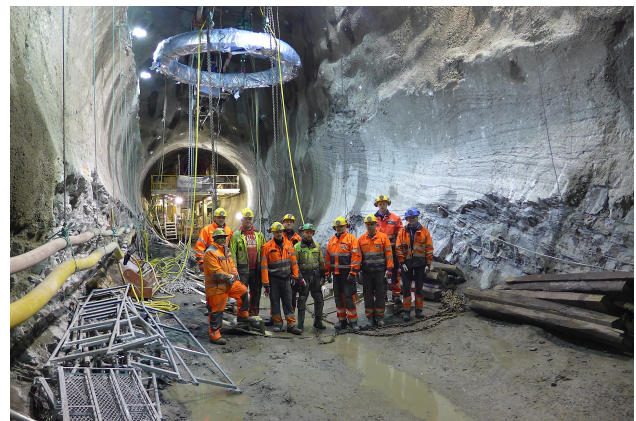
Figure 8. Workers during Main Bearing replacement (Anderson)
