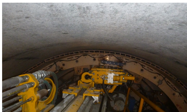
Figure 2. McNally slats in the shield and probe drill (Log)
