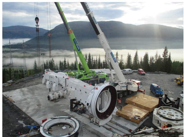
Figure 4. OFTA assembly at Røssåga (Gibson 2013)
