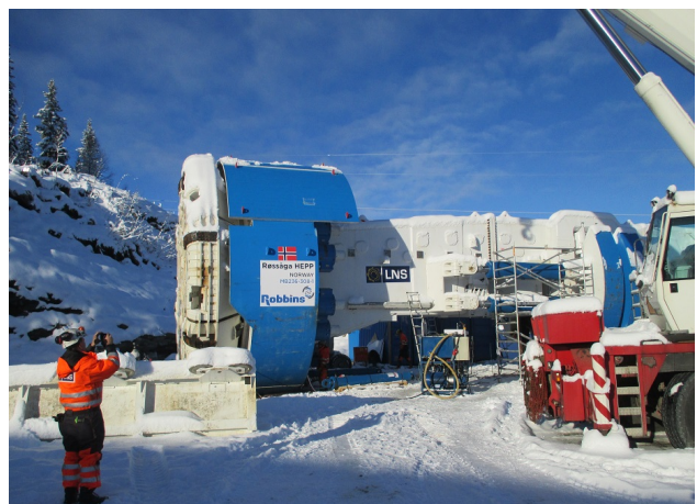
Figure 5. Assembled TBM in the snow (Solhaug 2013)
