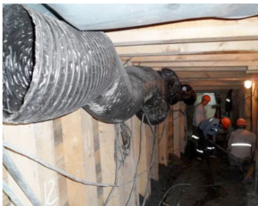
Figure 2. Bypass tunnel excavation
