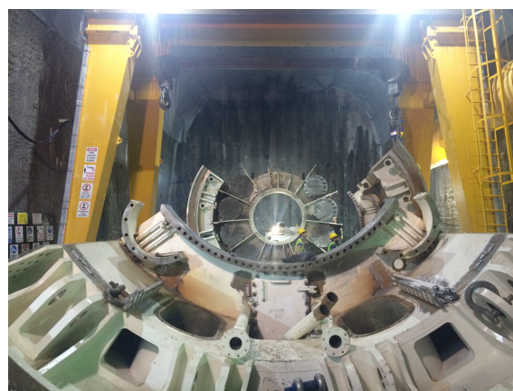
Figure 14. Assembly of the Gerede TBM in an underground launch chamber
