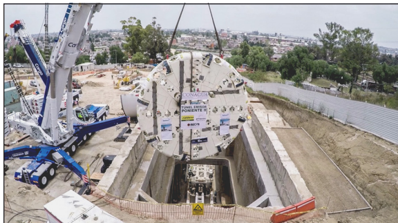
Figure 3. Cutterhead installation in a small launch shaft
