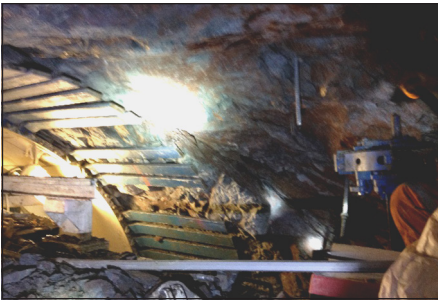
Figure 9. TBM excavation, overbreak with RMR = 32
