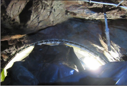
Figure 7. Sub-horizontal joints, RMR=42
