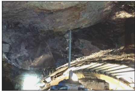
Figure 10. TBM excavation, overbreak with RMR = 32
