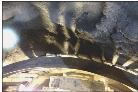
Figure 12. Ch. 13+862.31 and Ch. 13+861.50, support type IV
