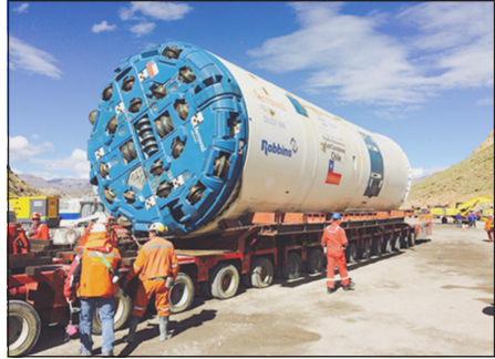
Figure 18. TBM being moved into launching chamber
