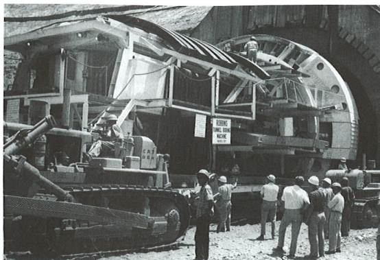
Pakistan's large-diameter Mangla Dam tunnel-boring machine used the first continuous conveyor to operate behind a TBM – a prototype that was developed by James Robbins
