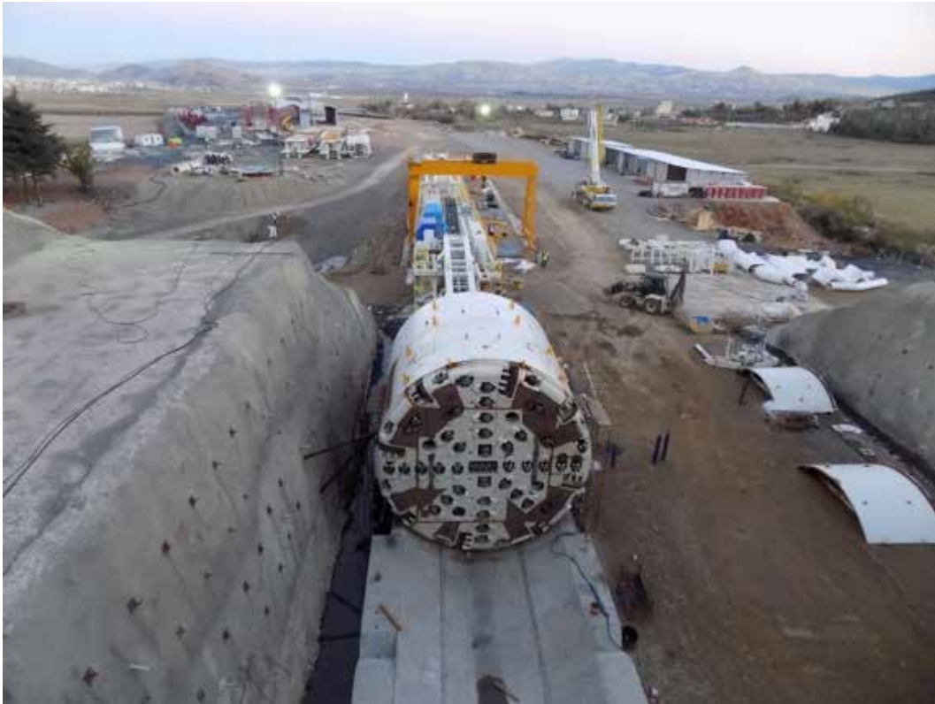
Figure 6. Onsite First Time Assembly of the Single Shield TBM.
