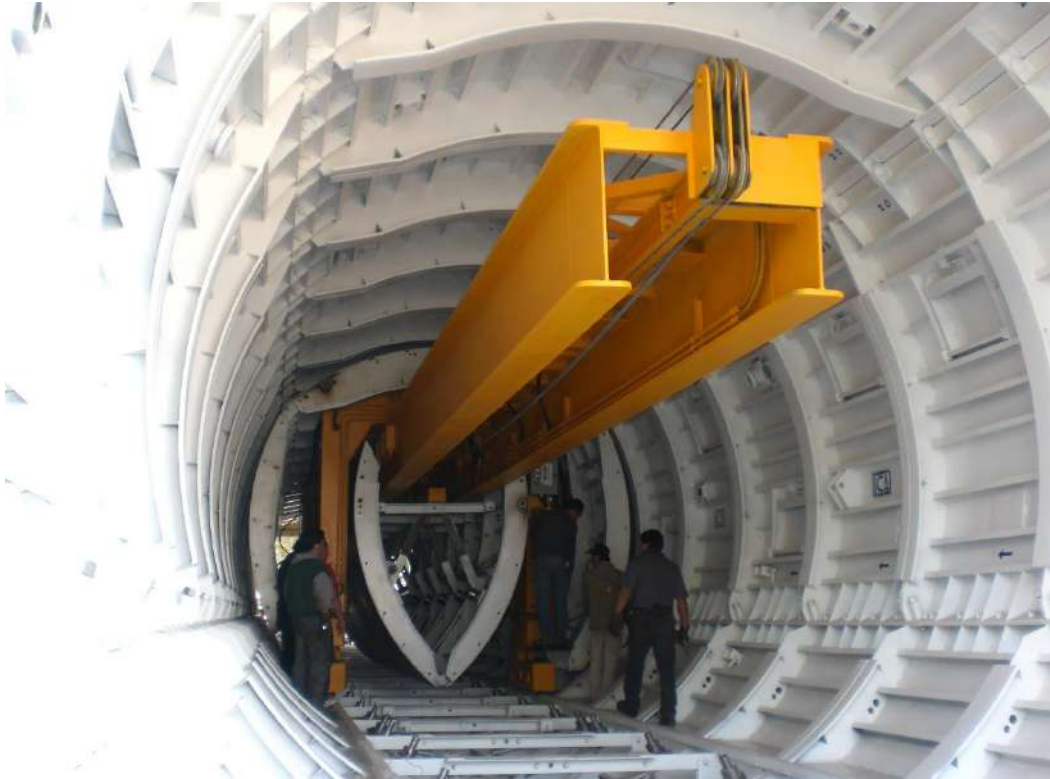
Figure 13. Cast-in-place concrete form.
