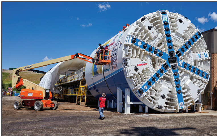
Figure 3. View of the OCIT TBM cutterhead
