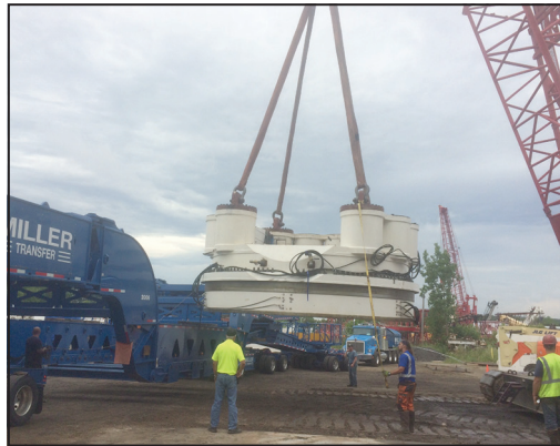
Figure 10. Transfer of the cutterhead support to a 19-axle truck
