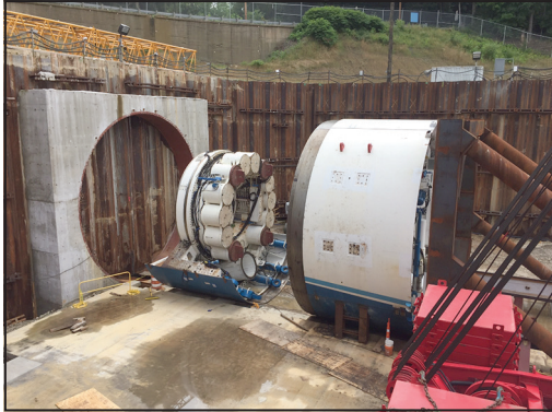
Figure 6. TBM assembly site and setup
