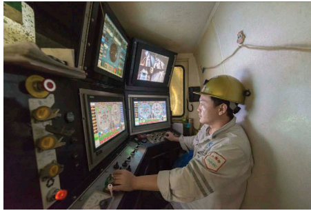
Figure 2. TBM data screens in operator's cabin.
