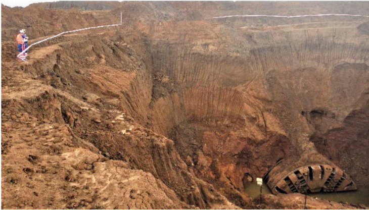
Figure 5. Excavation down to the TBM.
