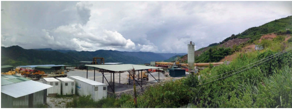
Figure 2. The Thuong Kon Tum job site.
