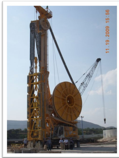
Figure 13. The hydro roadheader at shaft 20
