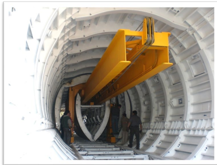
Figure 15. Cast-in-place form
