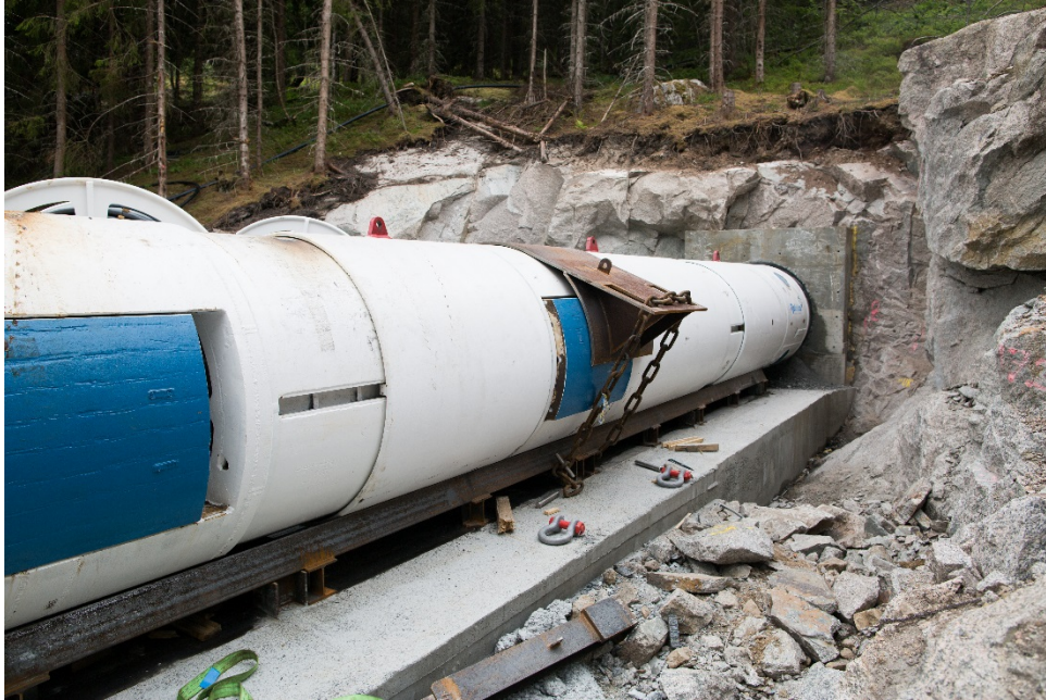
Figure 6. Double Shield Rockhead at Holen SHEPP (Photo: Endre Hilleren)
