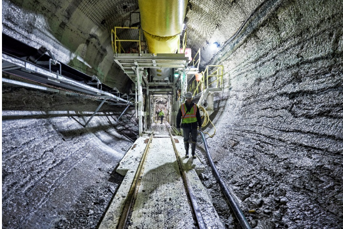
Figure 8. TBM excavation in limestone and shale rock
