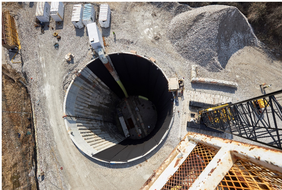
Figure 10. The 27 m diameter Jefferson Barracks shaft
