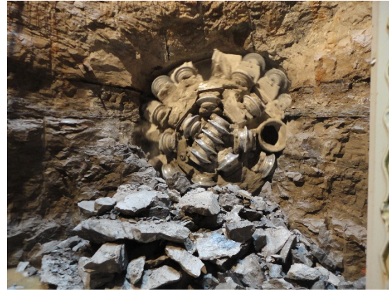
Figure 5. “Miss Colleen”, the Main Beam TBM for the Bi-County Water Tunnel
