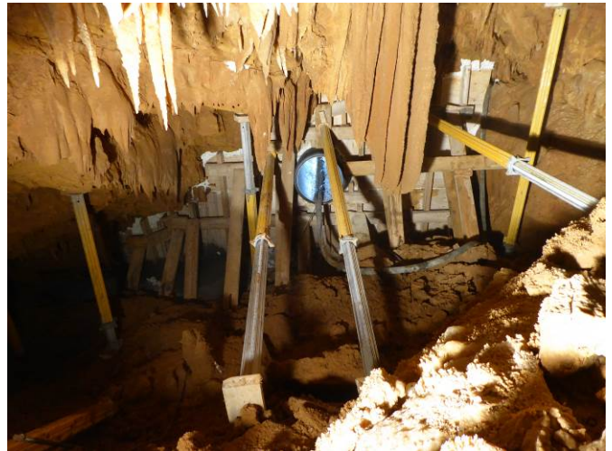
Figure 5 Wall of concrete erected to provide gripper support for TBM
