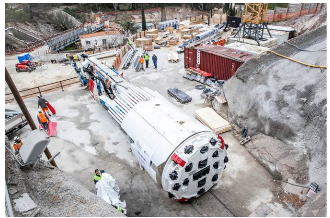
Figure 2 Robbins Main Beam TBM "Augustine" at site assembly
