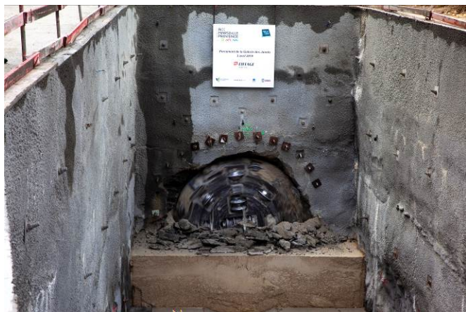
Figure 7 Machine breakthrough in April 2019
