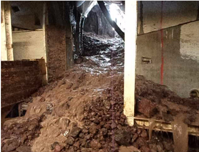
Figure 2 Of the three standard Double Shield TBMs used to originally bore sections of the tunnel, two became irretrievably stuck or damaged amid massive mud and water inflows
