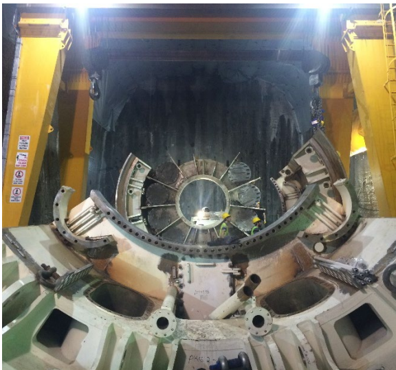
Figure 10 TBM assembly in the chamber
