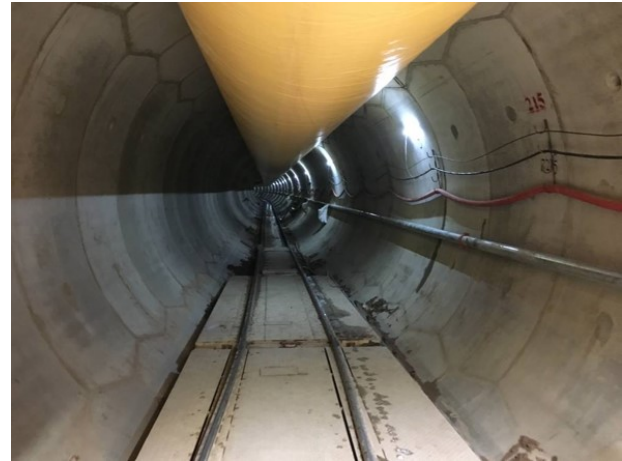
Figure 10. Completed lined tunnel section for BBDMP
