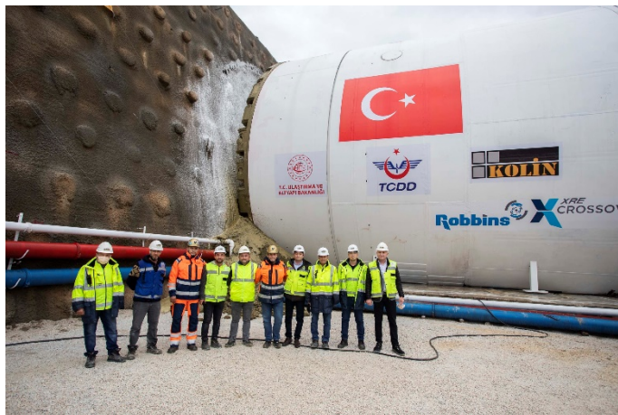
Figure 5. Ankara-izmir HSR Crossover XRE TBM
