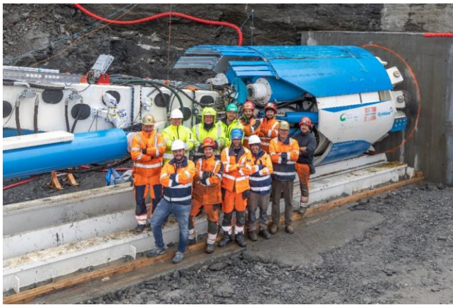
Figure 8. TBM ready to start boring Salvasskardelva (Photo: Kalle Punsvik)
