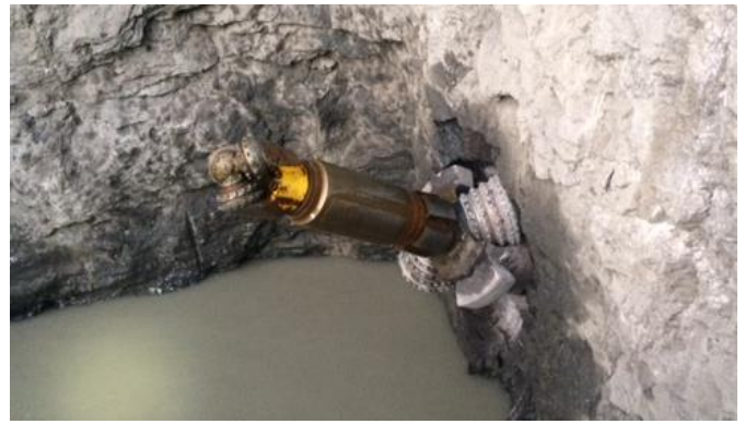
Figure 4. Norhard breakthrough with pilot hole on Grytendal project (NGK, 2019)
