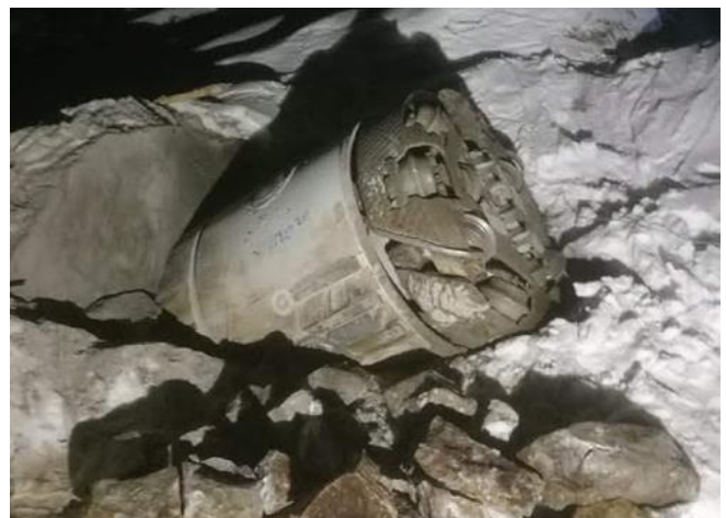
Figure 7. Breakthrough at Holen SHEPP (Photo: Hardanger Maskin AS)
