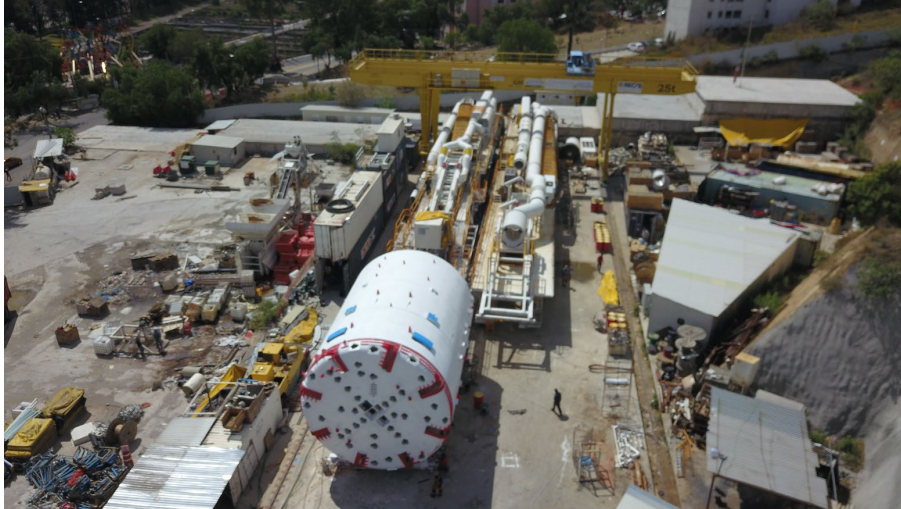
Figure 8. The Ashbridges TBM during the virtual machine acceptance in Mexico.
