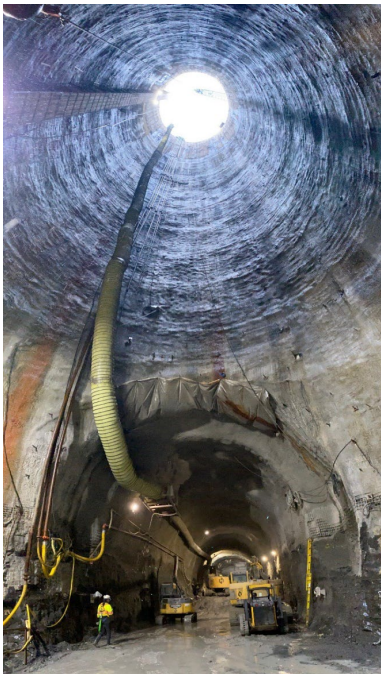
Figure 9. Starter tunnel at shaft bottom and cutterhead being lowered down shaft
