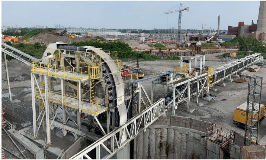
Figure 10. Project site at the surface with continuous conveyor configuration.
