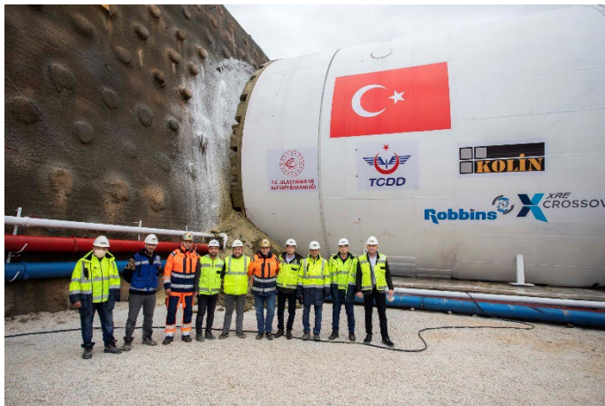
Figure 8. Ankara-Izmir HSR Crossover XRE TBM
